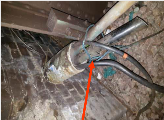
Cement pipe protruding from station platform.
